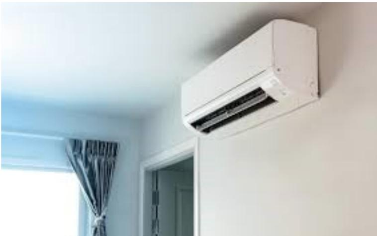
**Figure 1: Wall-mounted split unit type air conditioner**
